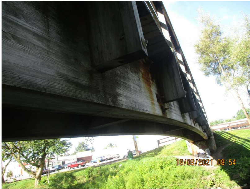
Figure 27 : Exterior Face of Girder (Typ.)
