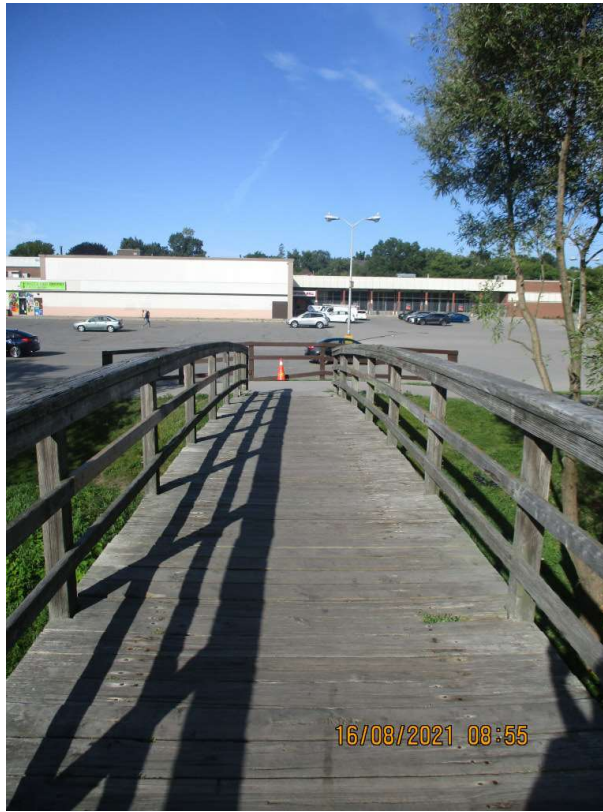
Figure 3 : Pathway Looking West
