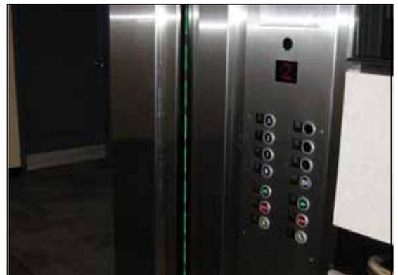
Elevator sensor door and floor registration buttons.
