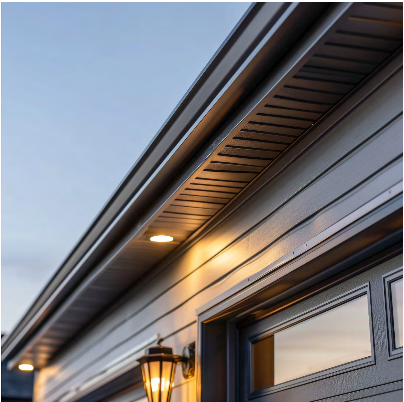
Figure 2 Soffit Lighting Example, Closeup
