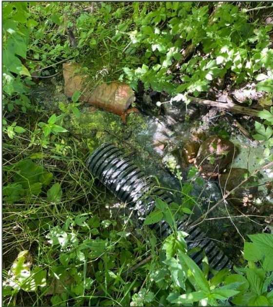
Photo 11: Tile Drainage terracotta pipes, corrugated pipe and stagnant foul water outlet
