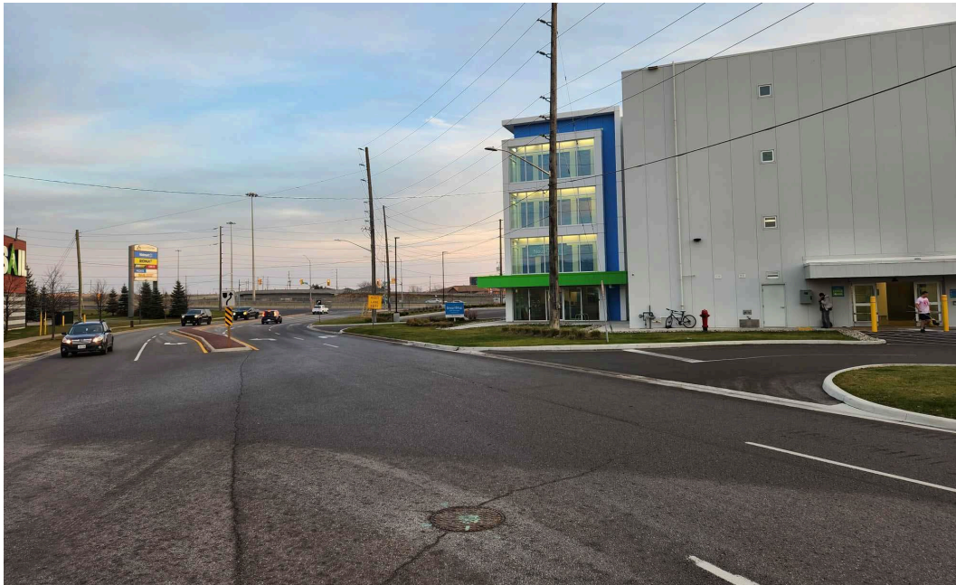
Figure 12 – Fox St. looking south towards Champlain Ave., SmartStop Self Storage at right
