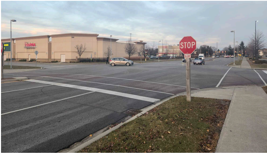
Figure 13 – Intersection of Laval Dr. and internal access road, Smart Centres Plaza, looking east towards Stevenson Rd. S.
