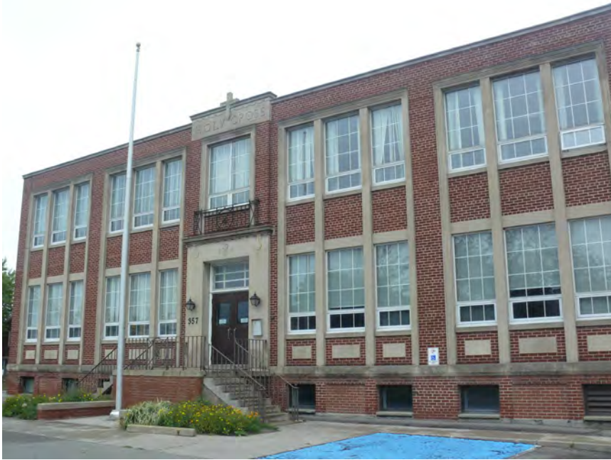
1. West Façade, August 2008
