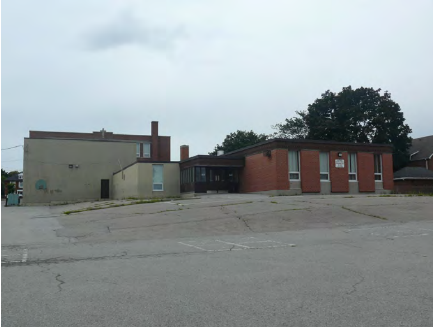
3. East Façade, August 2008
