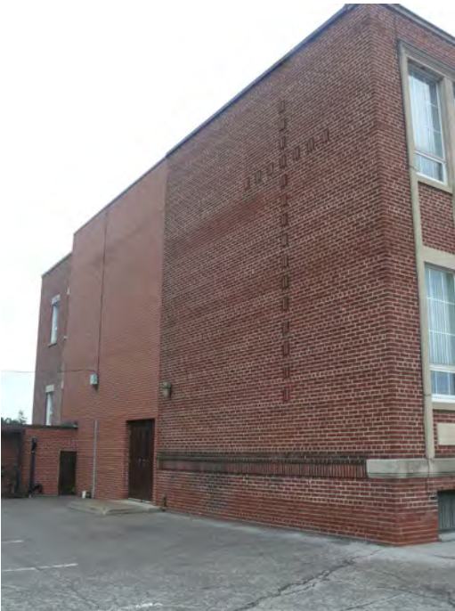
4. North Façade, August 2008
