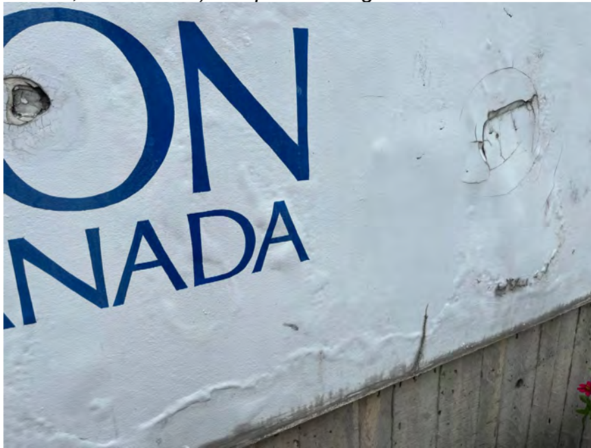
Figure 3: "Famous Oshawa Generals" (Paul Ygartua, 78 King St. West) – Streaks, cracks and water damage
