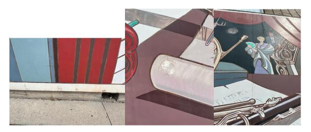
Figure Fourteen: "Borsberry Music Hall" (Brian Romagnoli, 31 Celina St.) – Water damage and discoloration from air conditioning
