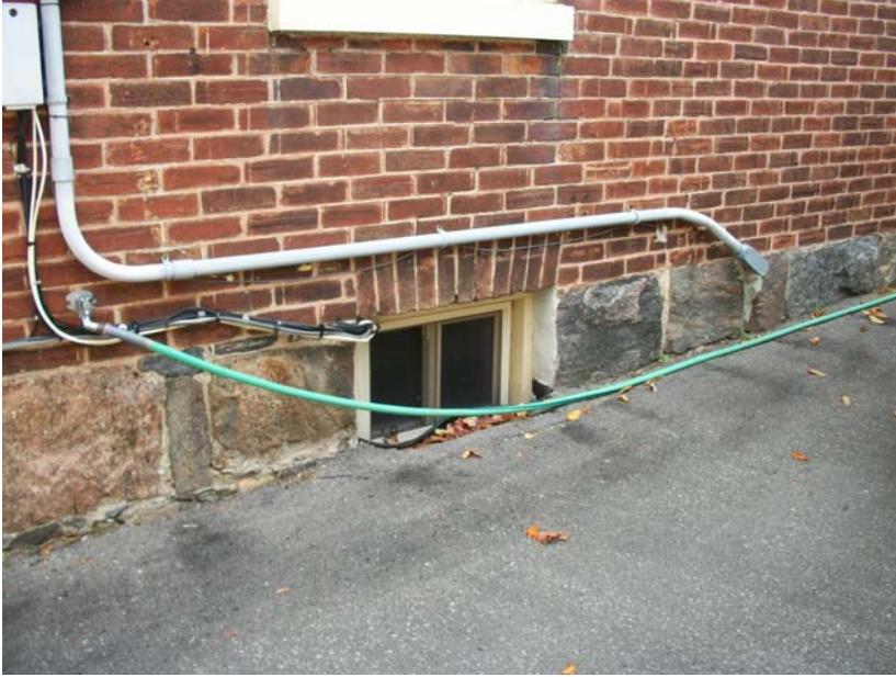
Basement Window, 442 King Street East, September 2010
