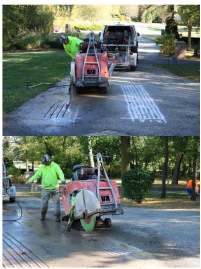
Saw cut each line to achieve at least a %" wide groove to fit a snow melting cable in. Multiple blades may need to be used to accomplish a wider cut. Test with a shorter cut first and use a cable to see if it fits in. Cuts need to be at least 1-½" deep, per National Electrical Code, and the cable should not run deeper than 2-3" from the surface to ensure proper performance. Plan a wider cut of about 9/16" or more for the 6" long
