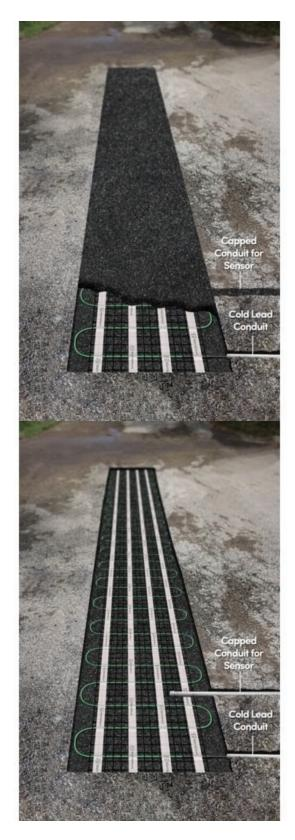
If you're installing a snow melting system for tire track coverage during a retrofit installation, an alternative trenching method may be used. Remove 2-3" of the top
