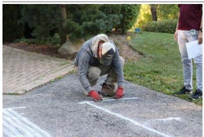
Prior to beginning any digging, we suggest contacting a local utility locating/marking firm to make sure your project won't run into any gas, water, or electrical lines. Once that's done, you'll want to start with locating the area to be heated and then, marking the cable layout in that area according to the SmartPlan.
