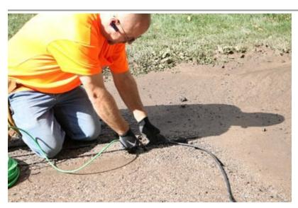
In this project, two separate heating cables (one in each tire track) are set up so that they 'begin' on the same side. This allows for one junction box to carry power to the cables
