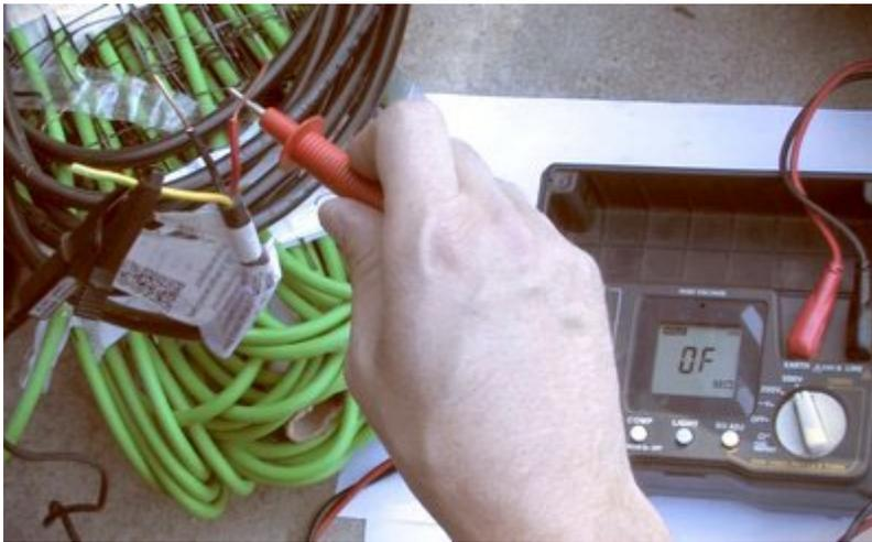
Testing your snow melting system with an ohmmeter and megohmmeter at every stage of installation will allow you to be certain that the heating element is functioning properly.
