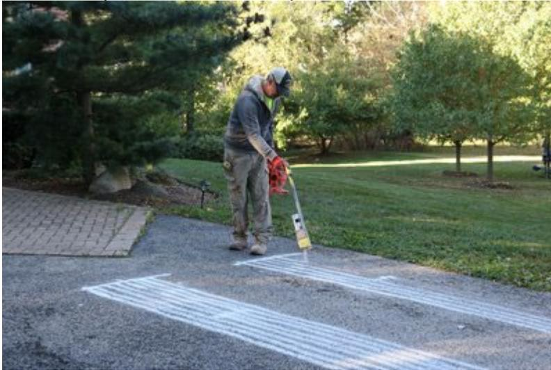
**Pro Tip:** While the chalk marking string is on the surface, spray the spray paint over the string to mark the position of the saw cuts. That will prevent the line from washing away and will provide a clear identification to ensure evenly-spaced and straight cuts.
