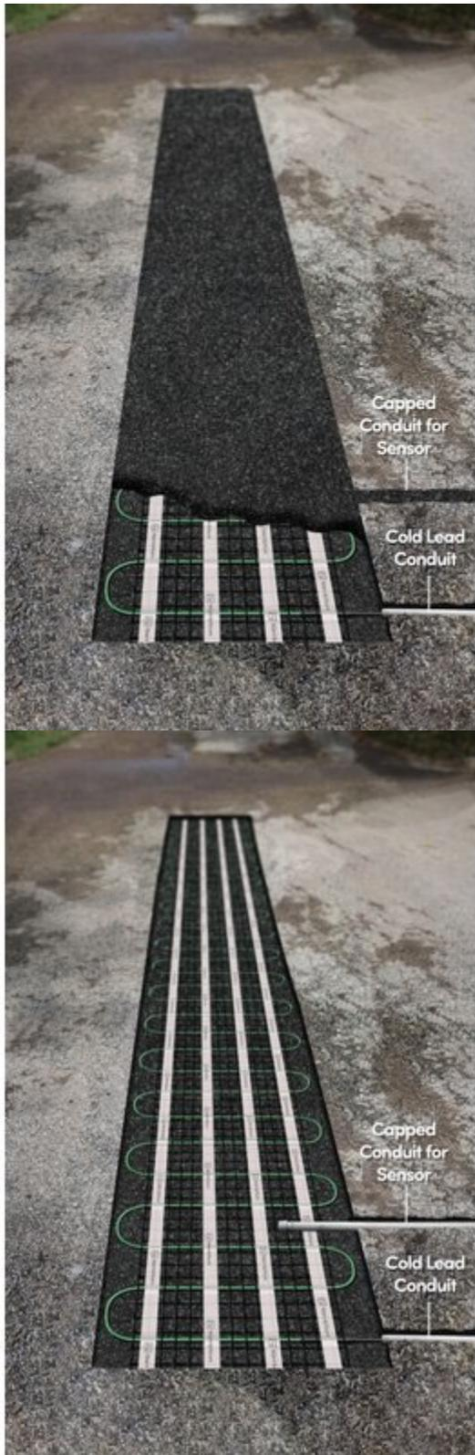
If you're installing a snow melting system for tire track coverage during a retrofit installation, an alternative trenching method may be used. Remove 2-3" of the top
