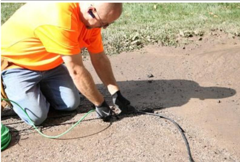
In this project, two separate heating cables (one in each tire track) are set up so that they 'begin' on the same side. This allows for one junction box to carry power to the cables.
