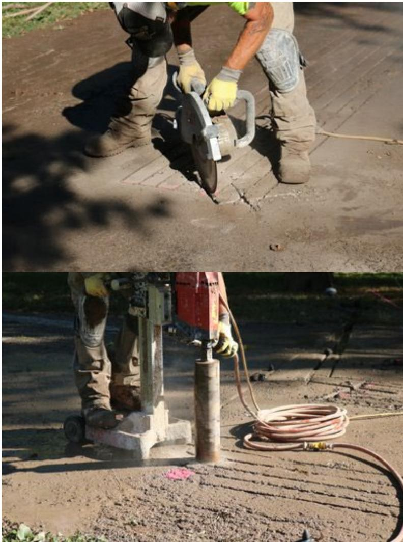
Round the corners of cuts to allow smooth cable placing in the U-turns. This can be accomplished by making additional 45° cuts at the U-turns or doing a core drilling with a core drill bit with a diameter matching the cable spacing (typically 3"). Please note that core drilling will require much more filler than the saw cut method will.
