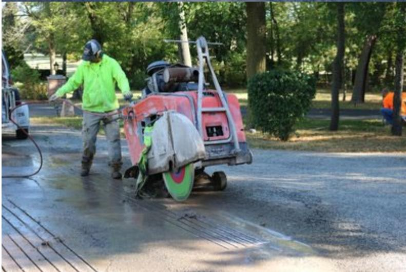
Saw cut each line to achieve at least a  $\frac{3}{8}$ " wide groove to fit a snow melting cable in. Multiple blades may need to be used to accomplish a wider cut. Test with a shorter cut first and use a cable to see if it fits in. Cuts need to be at least 1- $\frac{1}{2}$ " deep, per National Electrical Code, and the cable should not run deeper than 2-3" from the surface to ensure proper performance. Plan a wider cut of about  $\frac{9}{16}$ " or more for the 6" long
