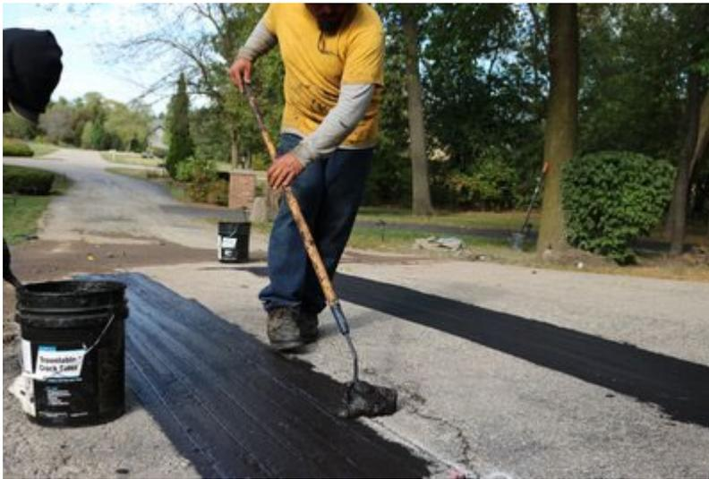
Fill all cuts with hot asphaltic sealer for asphalt retrofits, or expansion joint sealer (SikaFlex or similar) for concrete retrofits. Make sure this step is done in accordance with the filler manufacturer's recommended procedures.
