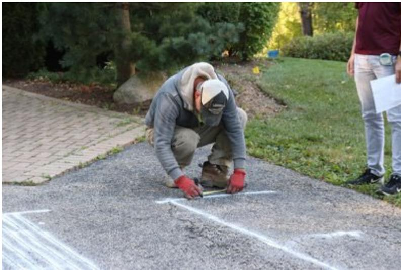
Prior to beginning any digging, we suggest contacting a local utility locating/marketing firm to make sure your project won't run into any gas, water, or electrical lines. Once that's done, you'll want to start with locating the area to be heated and then, marking the cable layout in that area according to the SmartPlan.
