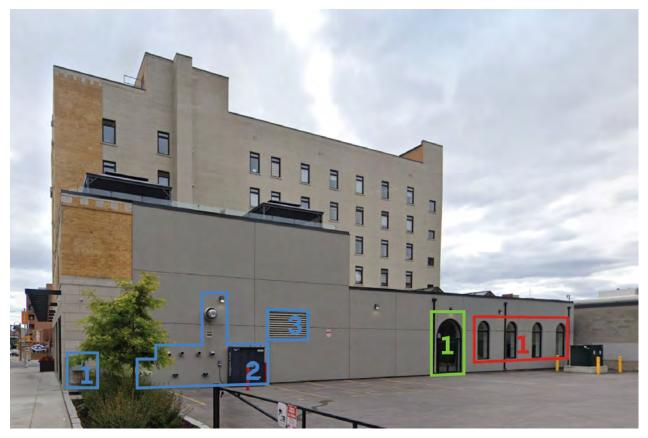
Blue: Electrical box, mechanical shafts, drainage systems and venting frille to be relocated Green: Existing glass door to be replaced a fire-rated door
