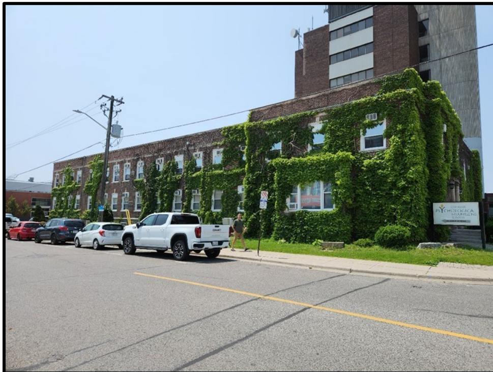
Image 4: East Elevation of 1948 East Wing of 117 King Street East (Photo taken June 19, 2023; Facing Southwest)
