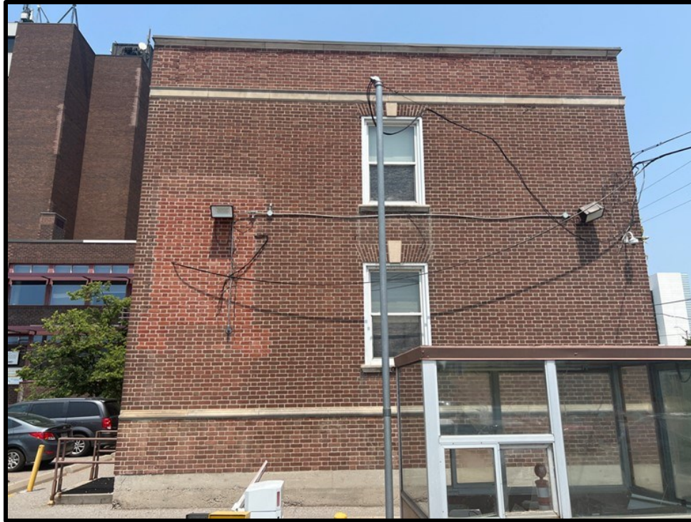
Image 5: South Elevation of 1948 East Wing of 117 King Street East (Photo taken June 19, 2023, Facing North)
