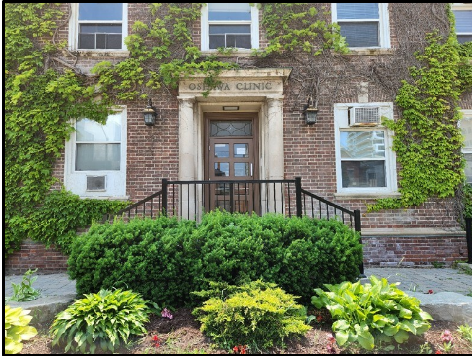
Image 3: Detail of Architrave and Recessed Entryway of 1948 East Wing (Photo taken June 19, 2023; Facing South)
