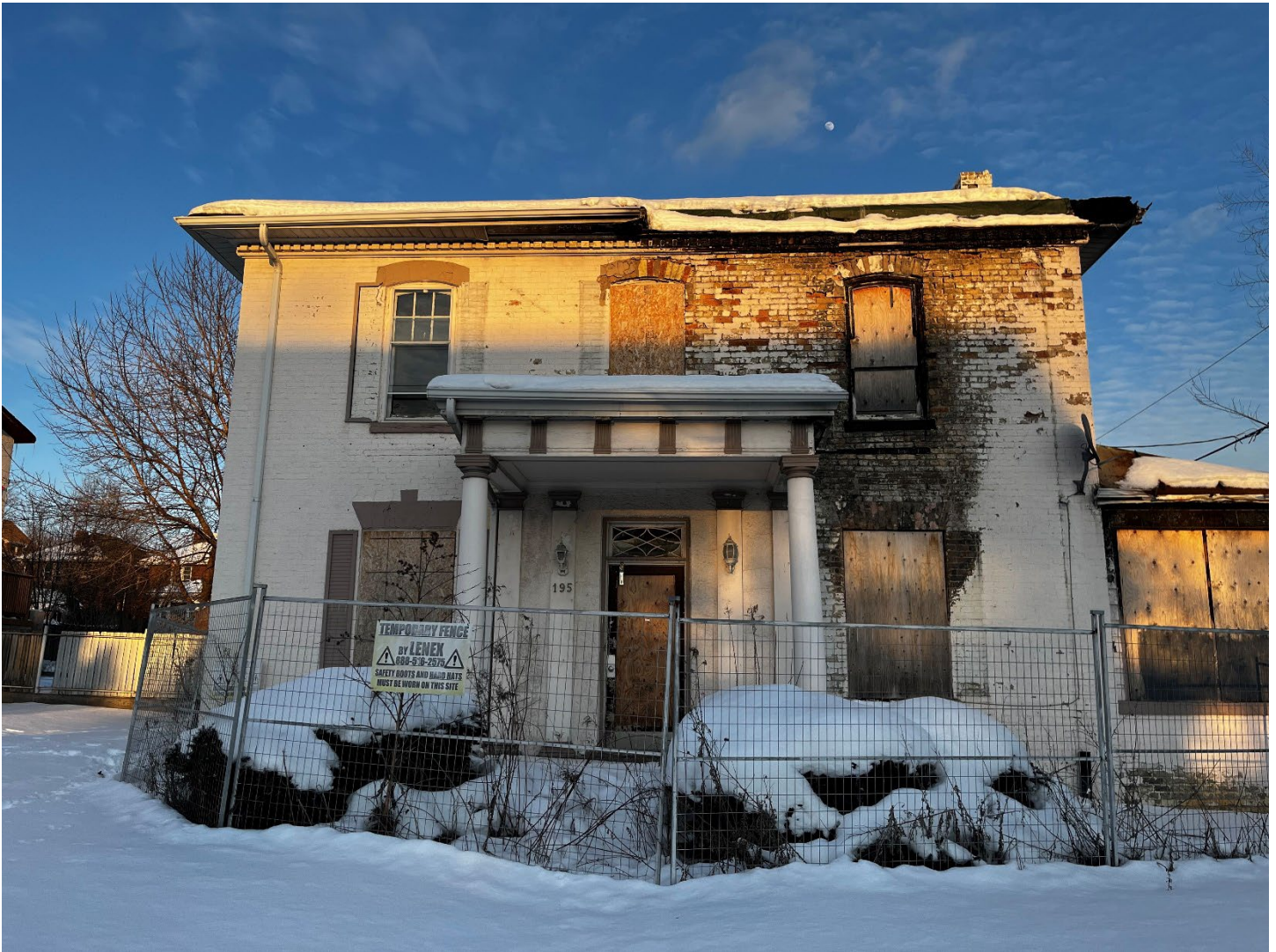
Figure 10 - Front of the building showing window treatments, fire damage, and structurally failing porch.
