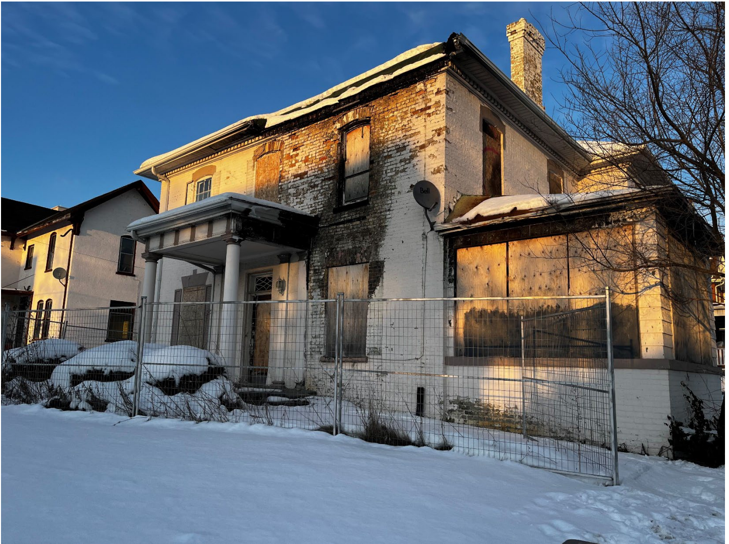
Figure 9 - Front of the building showing extreme fire damage and paint burning off the front.
