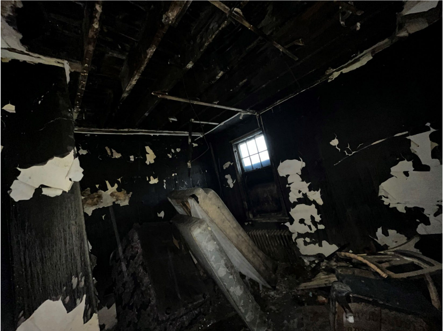
Figure 24 - Showing extent of fire damage, interior black from fire and burn.
