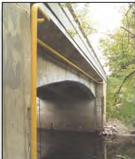
Attaching gas line on a bridge.
